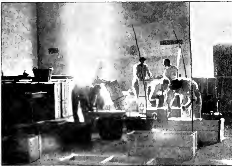
Coopering and Nailing the Cases.
